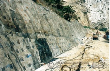
Temporary works support using Soil Nails
