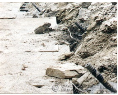
Soil Nails to resist subsidence
