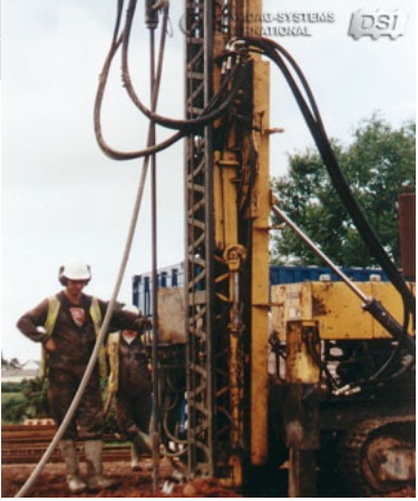
Simultaneous drilling and grouting
