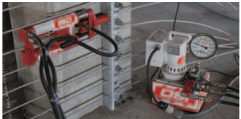
Backstressing of barrier cable.
