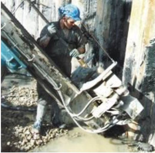
1. Drilling with a tungsten carbide button drill bit.
