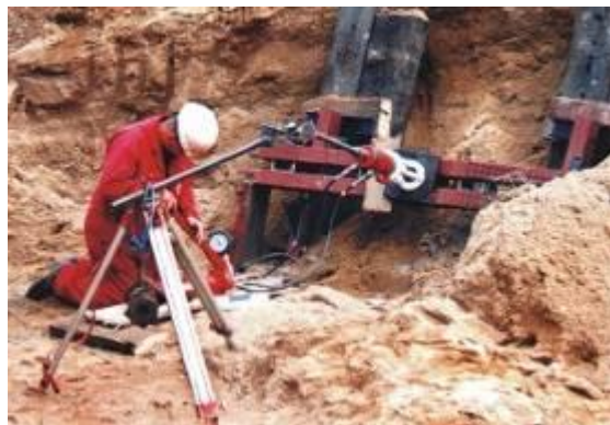
6. Testing of soil nails. Displacement is measured by a dial gauge (mounted independently), with load measured through a pressure gauge on the pump.
