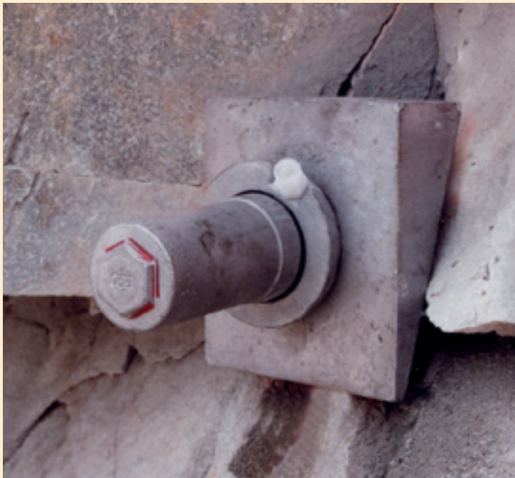
Anchor head with solid wedge plate and hemispherical seat (15°+12° angle compensation)
